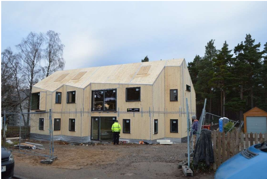
Figure 1. CLT house under construction
