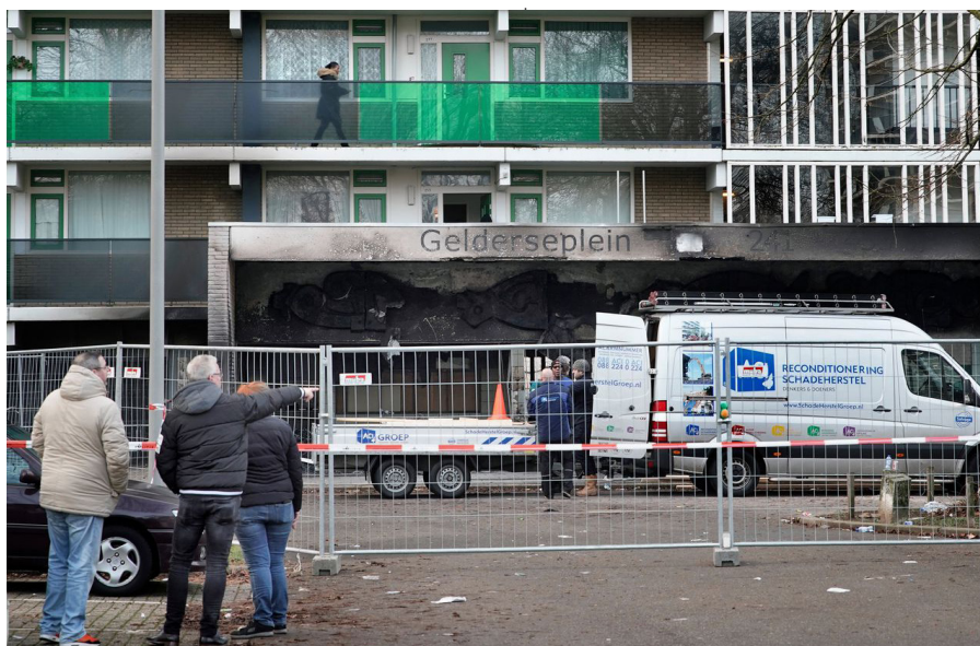
Figure 1: Entrance residential building Gelderseplein in Arnhem after the fire
