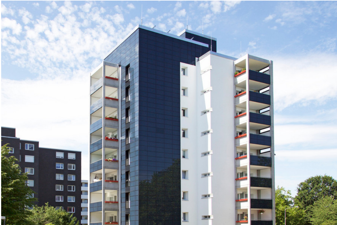
Figure 1.1: Residential building with BIPV facade in Bremen (Germany) [8]
