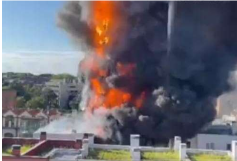
Woontoren in Milaan in brand (2021)
